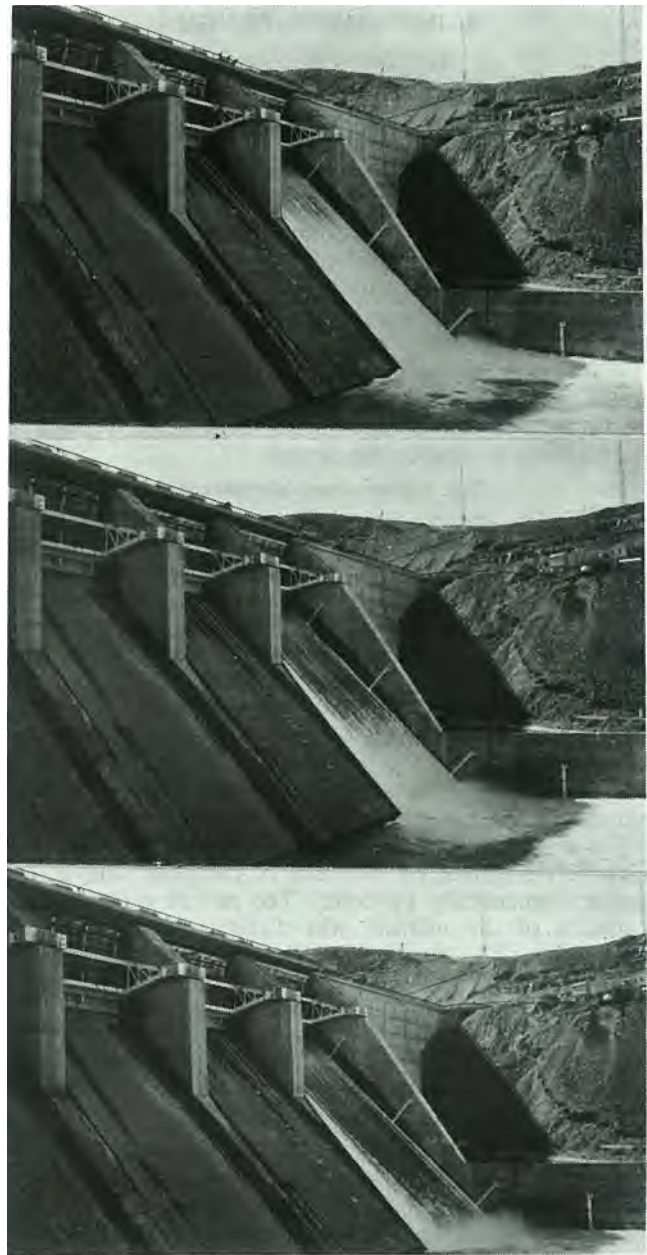
Fig. 2: Flow on Aviemore spillway. Top—gate opening 1 ft.; centre—gate opening 2 ft; bottom—gate opening 3 ft.
