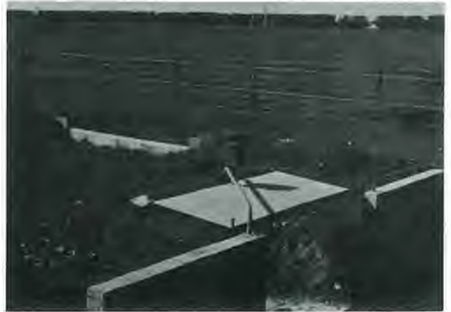
Fig. 1: Automatic irrigation dam and clock release mechanism.
