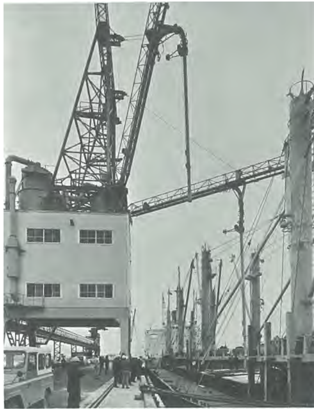
Fig. 2: Unloader on wharfhead.
