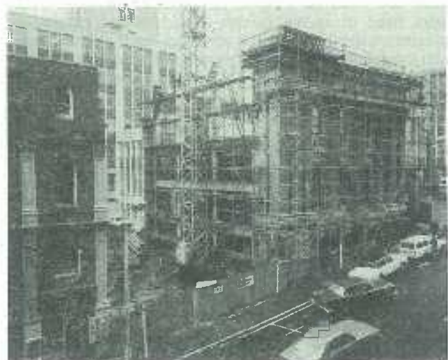
Fig. 3: New frame to east wall nearing completion; replacement of parapet commenced.
