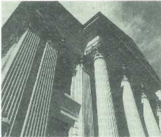
Fig. 2: Pediment and columns to front facade.
