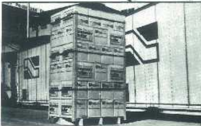
Above — The N.Z. Dairy Board bulk packages strengthened with Dimond angles
